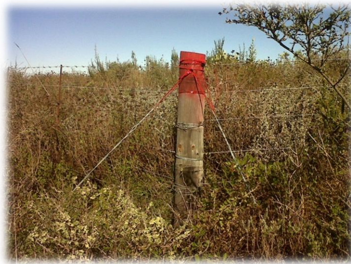
Figure 3: Wooden fence post beacon
